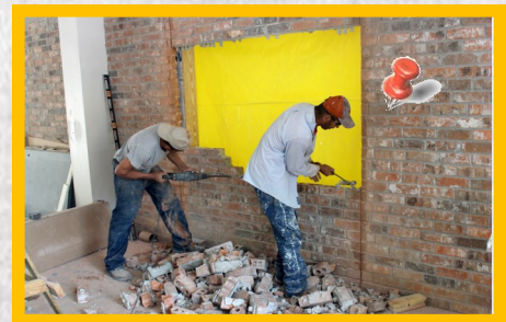
Workers Create a Passageway Between the Church and Education Building.
